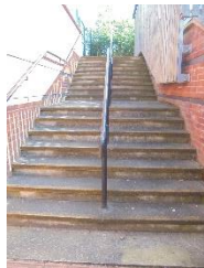
Stairs only in use by maintenance staff
